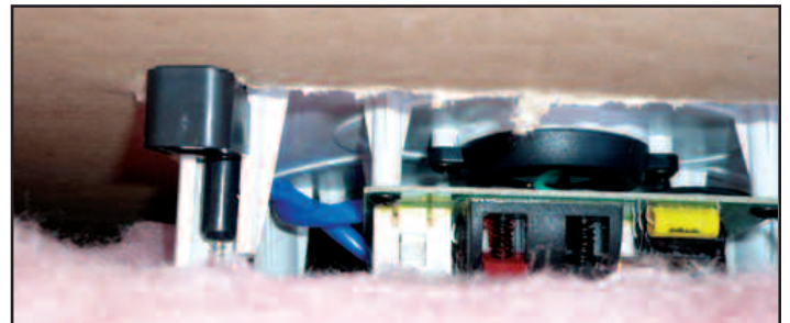
View of rotating cam after installation from inside the wall.
